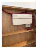
Fuses box inside White plastic, double socket Loose cable
