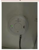
White plastic, carbon monoxide detector next to the boiler (top floor landing) New Tested and working
