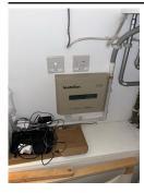
Heatmiser UH3, floor heating control panel to the back wall of the storage Good condition
