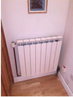
White painted radiator Good condition
