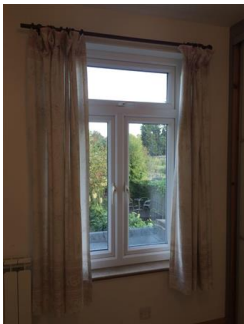
White UPVC frame, double glazed window with white lever handles with locks Good and working condition No keys attached
