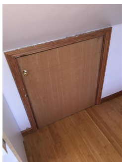
Wood, single door with knob handle, leading to small storage Good condition Paint marks to the frame
