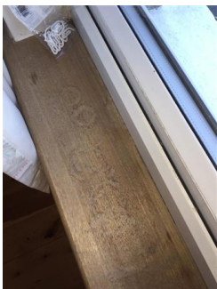
Wooden window sill Ring marks and stains
