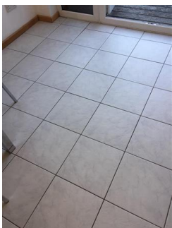
White and light grey, square tiles Few small chips in places Discoloured grout
