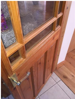
Light wood stained frame with clear glass panels, lever handle Marks consistent with age Slightly tarnished handle
