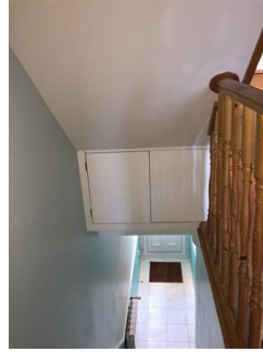
White painted double door storage above staircase Good condition
