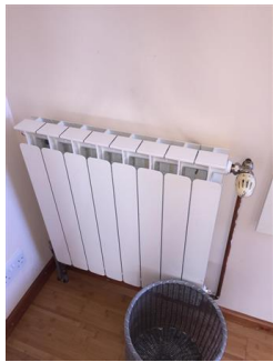
White painted radiator Good condition
