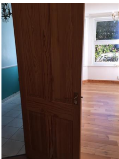
Light wood stained, panel door, brass lever handle Good condition overall Tarnished handle
