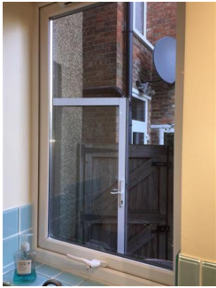
White UPVC frame, double glazed window with white lever handles with locks Good and working condition No key attached
