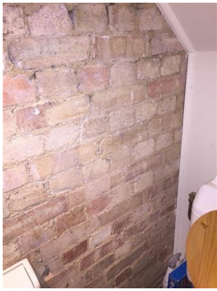
Old brick wall Good condition
