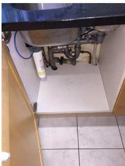
Internal view of sink cabinet
