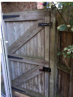
Wooden side gate with bolt lock to the top and chubb lock Good condition overall Weathered wood
