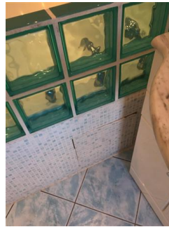
Blue glass tiles to divide basin and bath area
