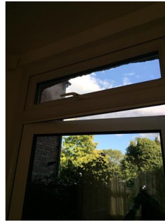
Window with lever handle above door Good condition
