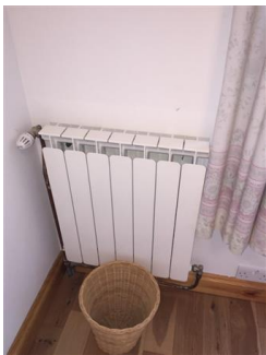
White painted radiator Good condition
