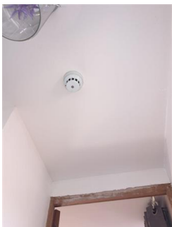
White painted ceiling Good condition White plastic heat and smoke detector to the top floor Good and working order
