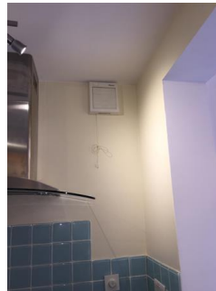
White plastic extractor fan with pull cord Tested and seems not working or not connected
