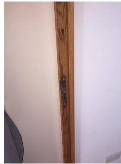
Light wood stained door frame Good condition overall
