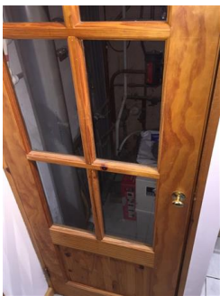
Light wood stained frame with clear glass panels, brass knob handle, leading to storage with boiler and water filter Marks consistent with age
