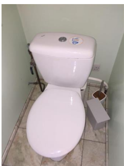
White wc with white plastic toilet seat White ceramic cistern with chrome push button Good condition
