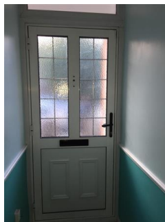
Internal view to match Good condition
