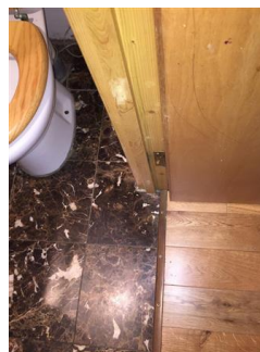
Marked frame to level Threshold in good condition
