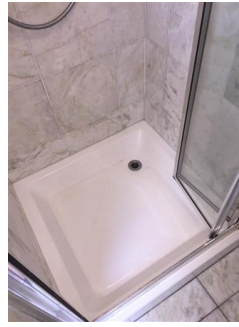
Built in shower cubicle with clear glass and chrome, foldable door, white base Good condition
