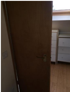
Light wood stained flat panel door, brass lever handle Good condition overall Tarnished handle
