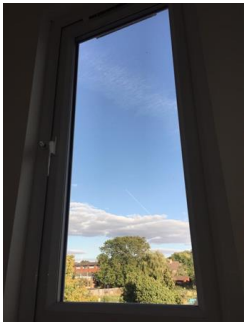
White UPVC frame, double glazed window with white lever handles with locks Good and working condition 1x key attached
