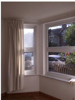
White UPVC frame, double glazed window with white lever handles with locks Good and working condition No keys attached
