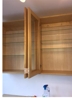
Internal view Good condition
