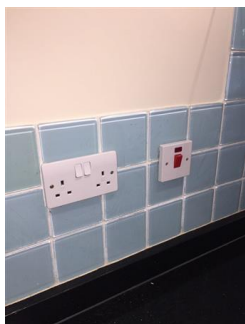
White plastic, double socket and single fuse Good condition
