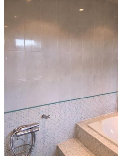
Blue mosaic tiles and light tiles to top Good condition
