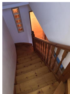
Wooden banister Good condition
