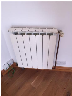
White painted radiator Good condition
