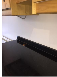
White painted walls Good condition
