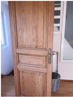
Light wood stained panel door, brass lever handle with chubb lock Good condition overall Tarnished handle
