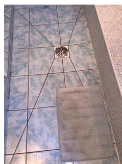
Wet area to match Good condition
