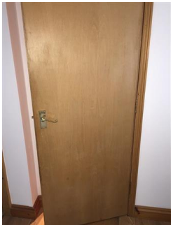
Light wood stained flat panel door, brass lever handle Good condition overall Tarnished handle
