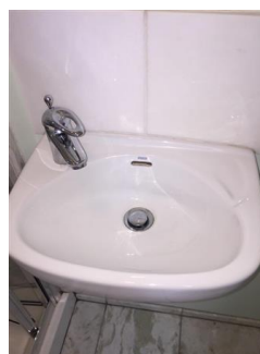
White, small basin with chrome pop up waste and chrome mixer tap Good and clean condition
