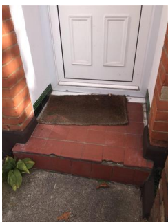
Red tiles to the step outside front door Chipped to edge Worn
