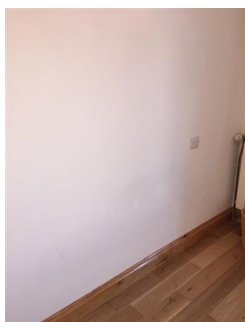
White painted walls Wooden skirting Good condition overall
