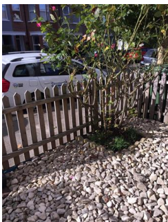
Wooden fence to the front Weathered
