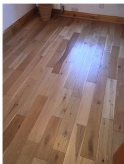
Light wood floor boards Good condition
