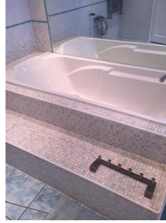
Raised tiles step to bath
