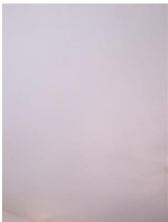
White painted ceiling Good condition
