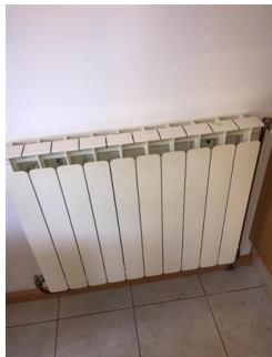
White painted radiator Good condition
