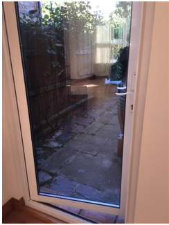
White UPVC frame, double glazed single door with white lever handle with cylinder lock, door leading to the rear garden Good and fully working order
