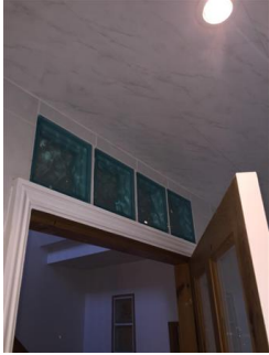
Blue glass tiles above door Good condition
