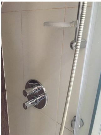
wall mounted chrome shower control, shower mount, flexible hose to shower head
