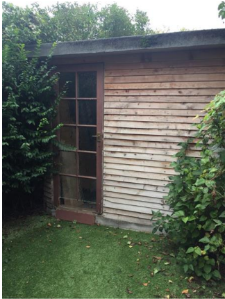
Shed, light wood, dark brown door with glass panels, gold lever handle, door not closing properly, cracked
